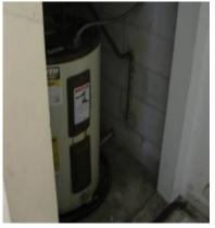
The largest energy savings came from replacing this 30-gal tank electric water heater with a 50-gal electric/heat pump hybrid water heater. The new water heater will save an estimated \$182 annually in energy costs. Only relatively minor modifications were required to fit the new water heater in the old unit's space.
